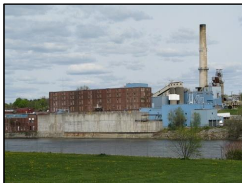
Former Scott Paper Mill
