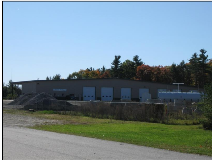
New Public Works Garage
